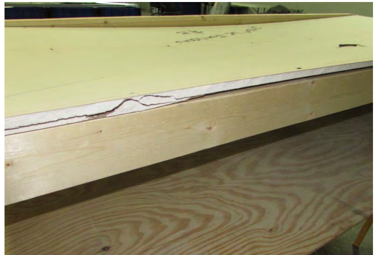
Test Sample #3 Failure
